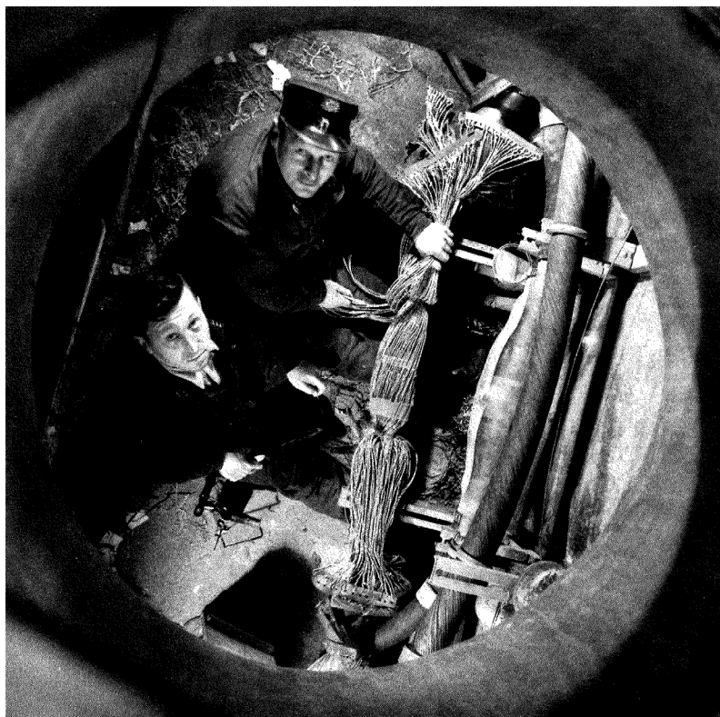
FIG. 4. Maintaining Hidden Infrastructure. Although the photograph showing PTT Workers maintaining underground cables is undated, editors included it in a 1941 commemorative volume celebrating the telephone workers' contribution to the Swiss Confederation. The image illustrates a vital yet often unseen aspect of their maintenance work while emphasizing its technical difficulty, with two monteurs working through a tangled bundle of wires. Considered in a broader context, the photograph presented underground cable maintenance as specialized technical labor essential to the operation of modern communications infrastructure. (Source: Bratschi, Fiers de servir .)
