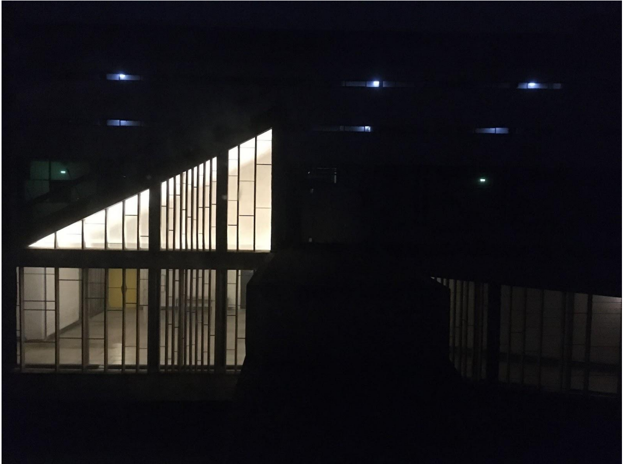
Figure 25: View of the atrium triangle with the posts on top of each other
