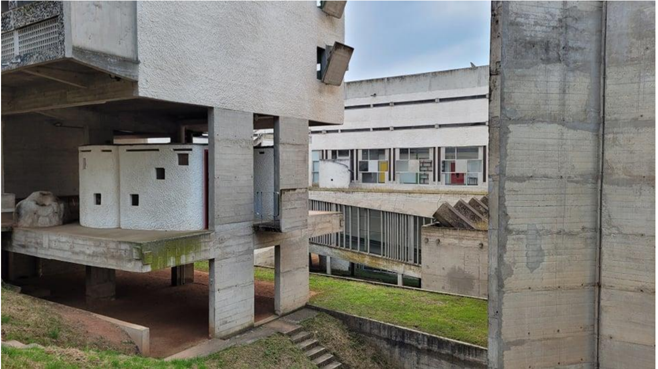
Figure 1: opening to the interior of the convent, near the entrance
