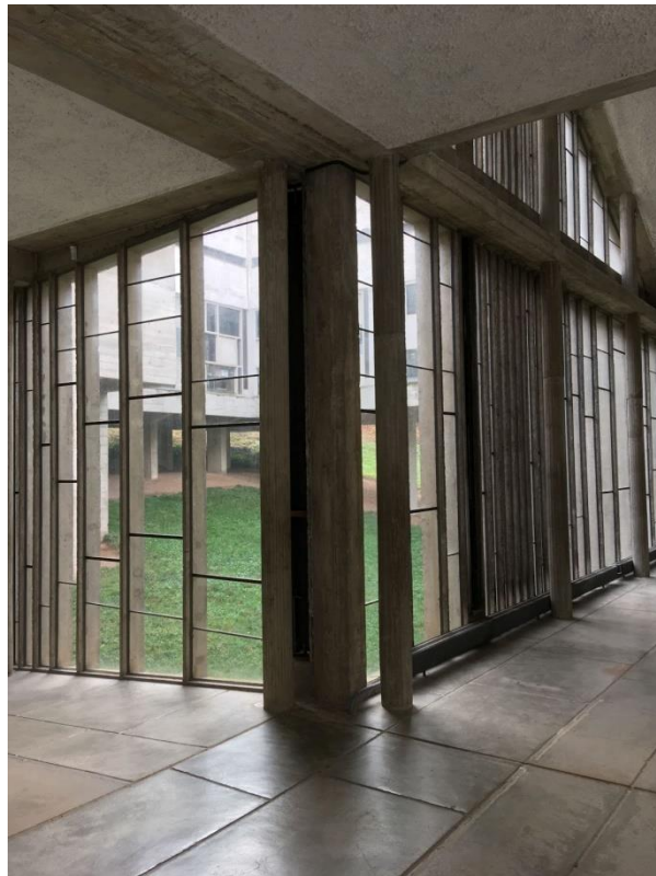
Figure 23: the corner between the “Grand” and “Petit Conduit”
