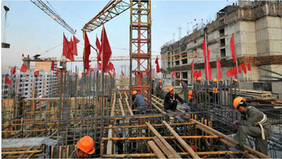
Figure 90. Mirae Street Development During Construction 251
