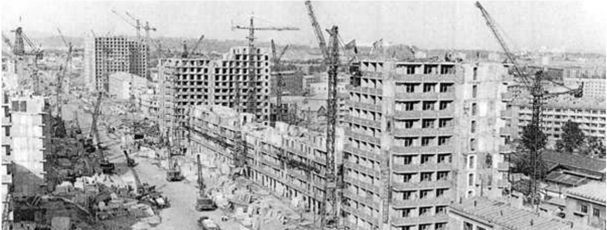
Figure 70. Ragwon Street Development during Construction 239
