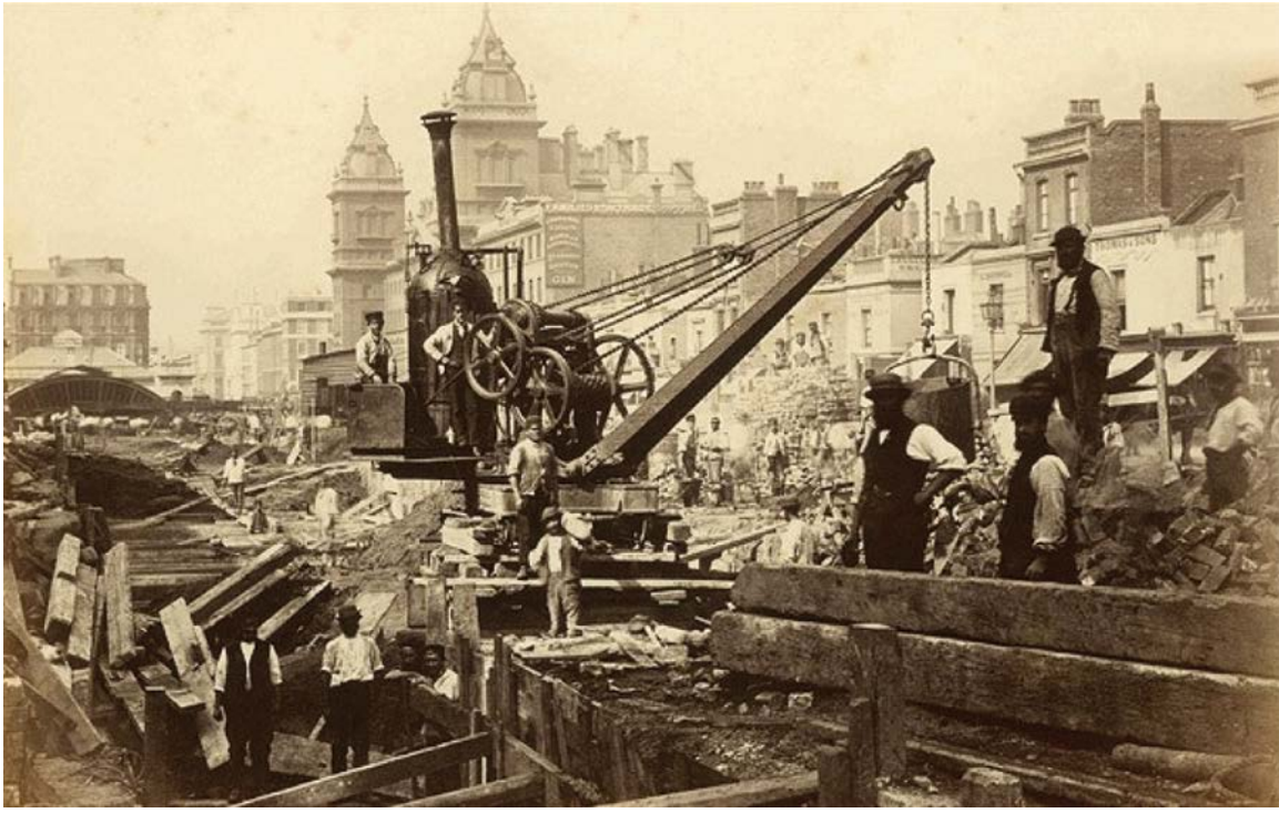
Figure 4. Capitalism meets the city: 1867 photograph by Henry Flather of the construction of the Metropolitan Line at Praed Street next to Paddington Station, forming part of London's new underground railway network (© Museum of London).
